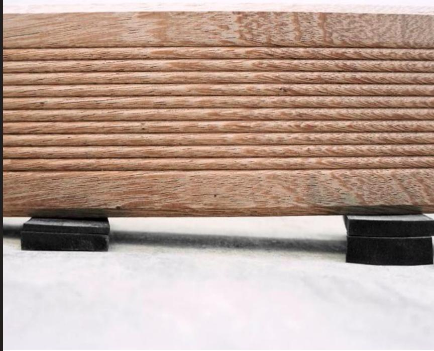
The **GUMO L** pads ensure optimum ventilation between the substructure and the substrate. Different thicknesses make it easy to compensate for differences in height, and several can be stacked on top of each other.
